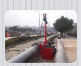
Do not remove joint from root for an additional 3 minutes. Do not stress joint for at least 10 minutes after removal from root.
